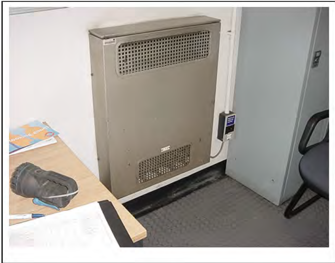
Figure 19: Material Strongly Presumed To Contain Asbestos
